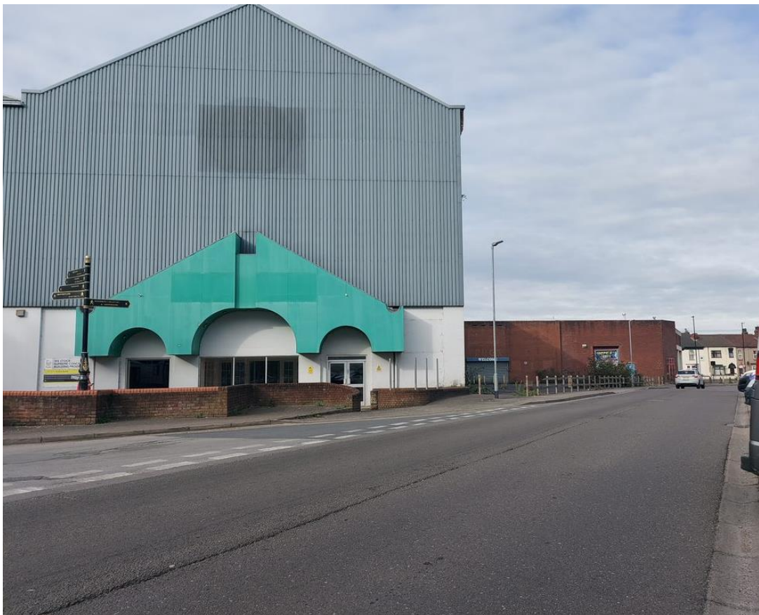
View west along Dunford Road
