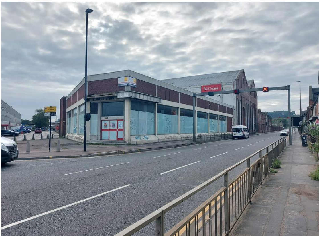
View from the footpath opposite the site
