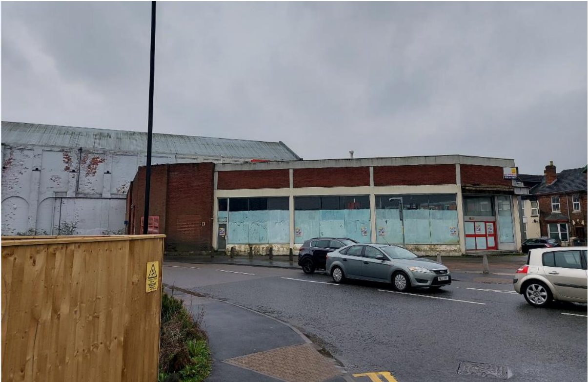
View from the corner of Kesteven street and Dunford Road junction
