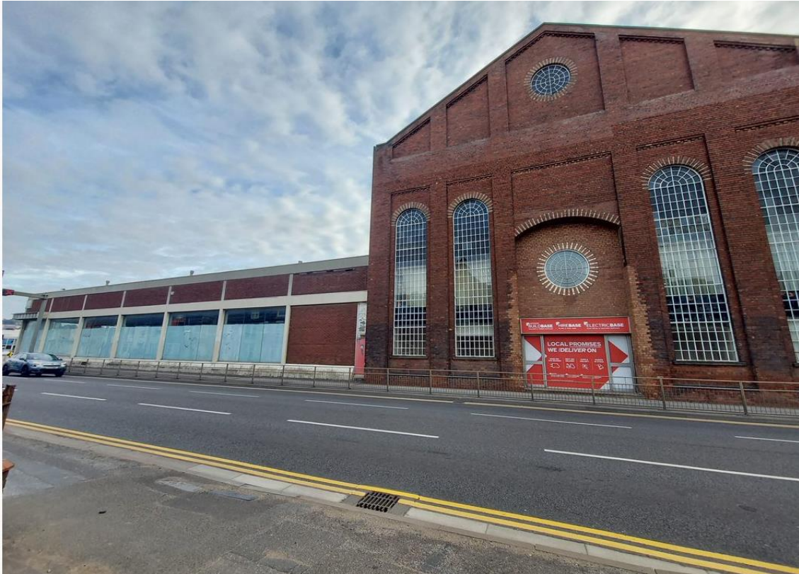
View from the footpath opposite the site
